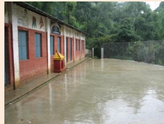
Concreting front area of school
