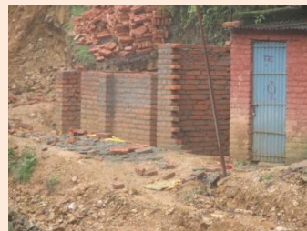
New school toilet block
