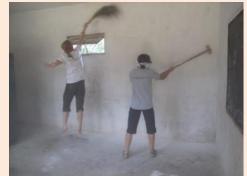
Preparing a classroom to be painted
