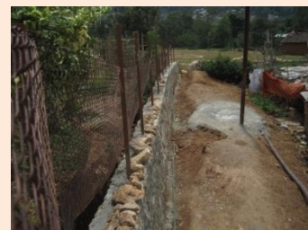
BFCH retaining front wall
