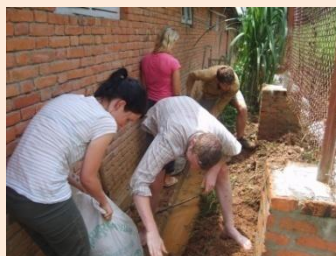
Sandbagging BFC's back wall
