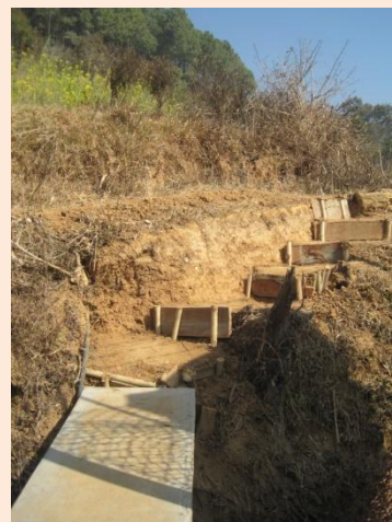
Bridge & steps for BFCH back gate
